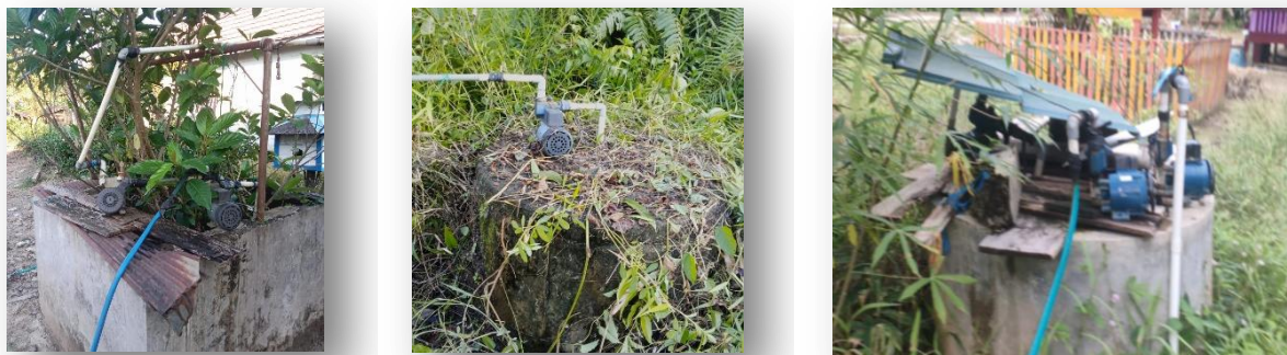
Figure 2 The actual condition of modified dug-well (combined with a water-pump or many water pumps). All wells are overgrown and does not meet the WHO criteria for protected well.
